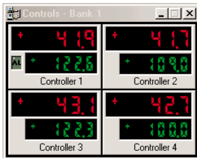
Controller Faceplates provide an operator view of alarm, PV and Setpoint.
